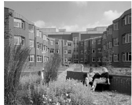
CoCo-Web remotely controlling heating systems in building complexes.
